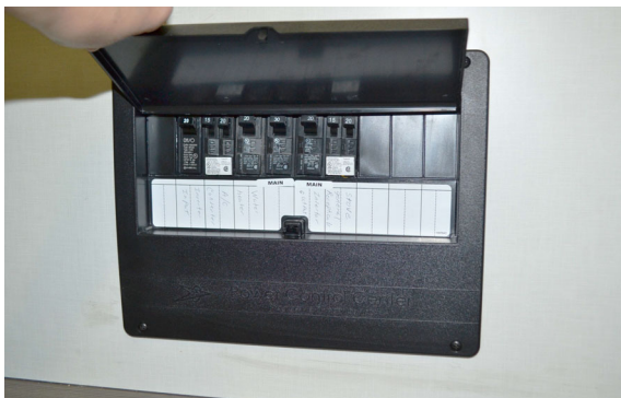
120-Volt Circuit Breakers -Typical View
